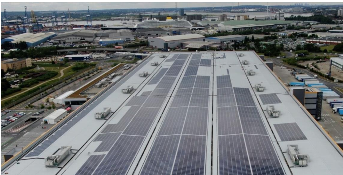
Amazon's Tilbury fulfilment centre: The building has 2 million sq. ft. of operating space and has been fitted with more than 11,500 modular solar panels, which generate the equivalent amount of electricity required to power UK 700 homes for one year.
